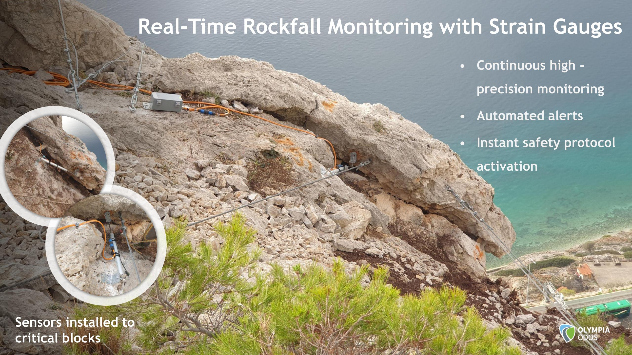
Sensors installed to critical blocks
