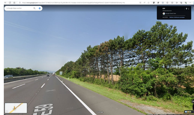
Example of downgrading <12.5m
