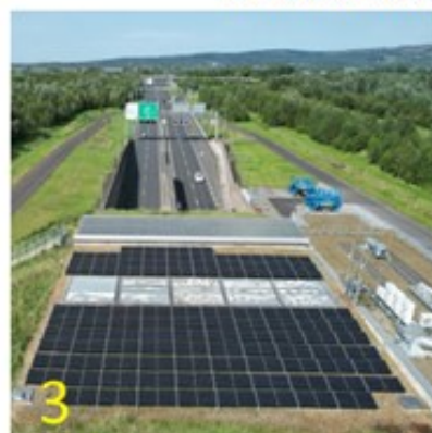
3. North Services Building
