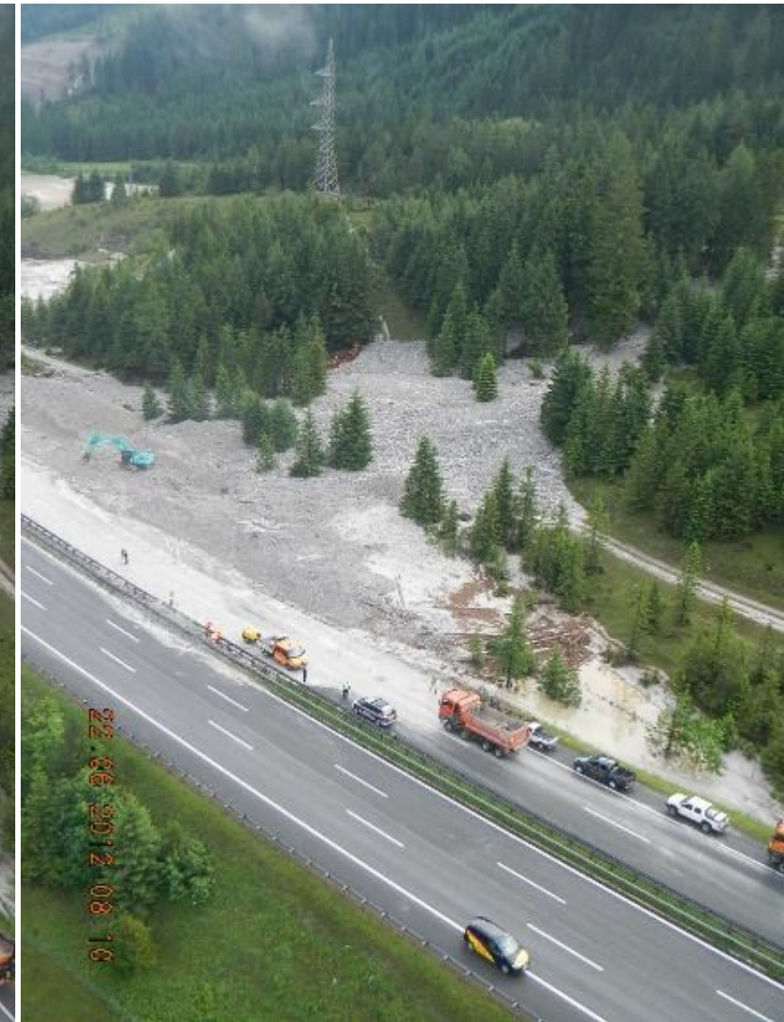
Gravel Landslide, A 10 Highway, 2012
