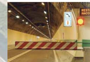
A particular and careful attention is to be paid to the design of tunnels and the respect of high safety standards. These standards are guaranteed both by structural features (e.g. dual-bore tunnel), and by management and emergency systems. Actually, tunnels are equipped with a large number of devices to control and regulate traffic, to communicate with users and to
